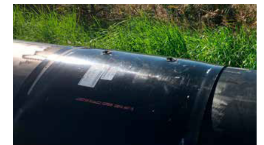
The barcode contains unique data on the joint type and dimension, and the resistance of the welding wires.
