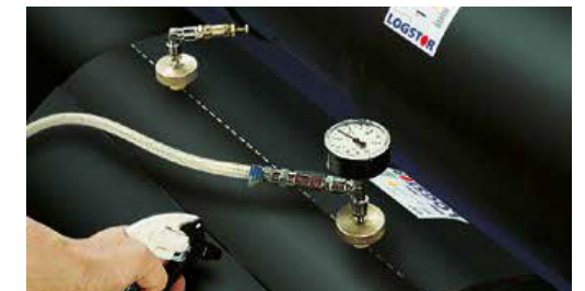
Leakage test before foaming.
