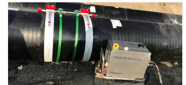
LOGSTOR WeldMaster with two welding units. PDA/LOGSTOR Connect for remote control of the welding process. The 2D barcode on the joint contains the necessary data for the welding process and is scanned with the PDA/LOGSTOR Connect.
